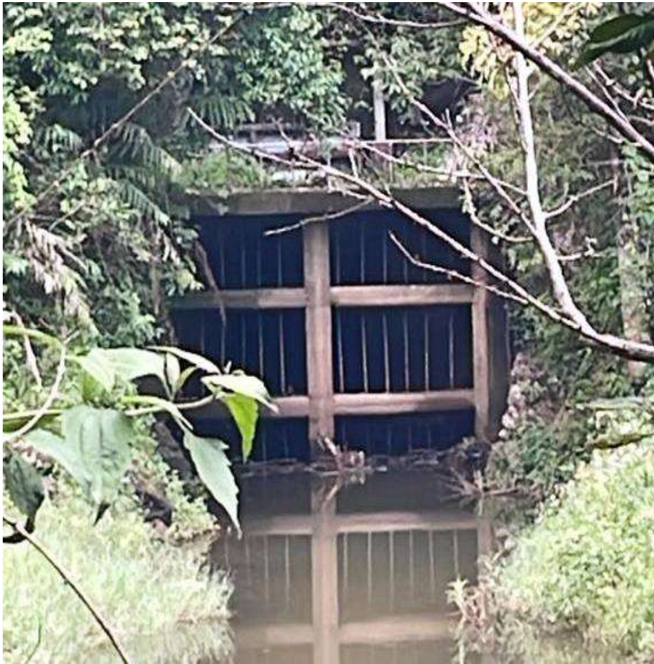
Fig 1.8 Kuttiyar Diversion Weir – Trash rack at Intake (Inlet)
