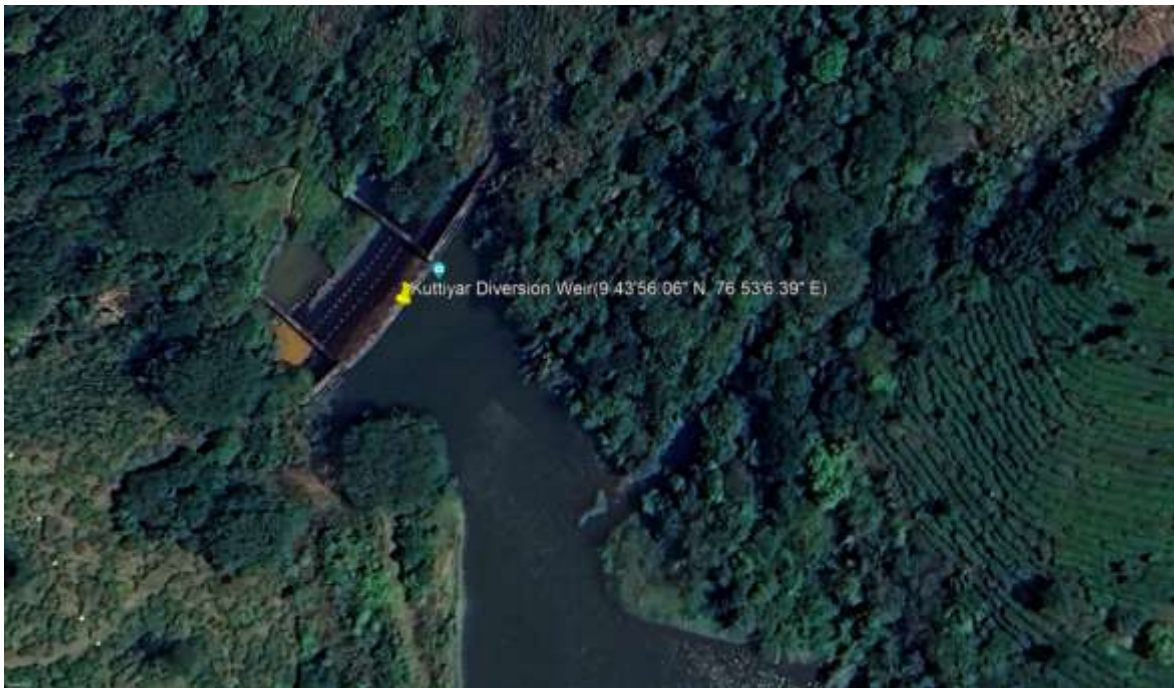
Fig 1.6 Kuttiyar Diversion Weir - Google view
