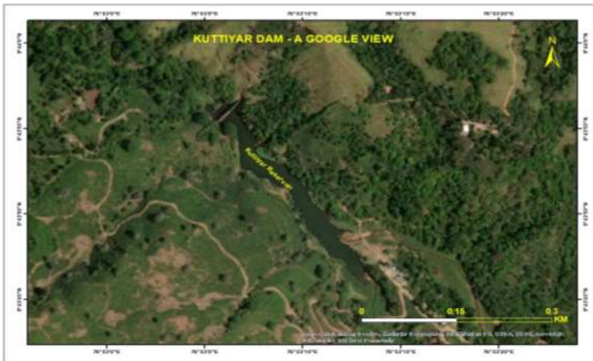
Fig 1.2 Kuttiyar Diversion Weir- Google View
