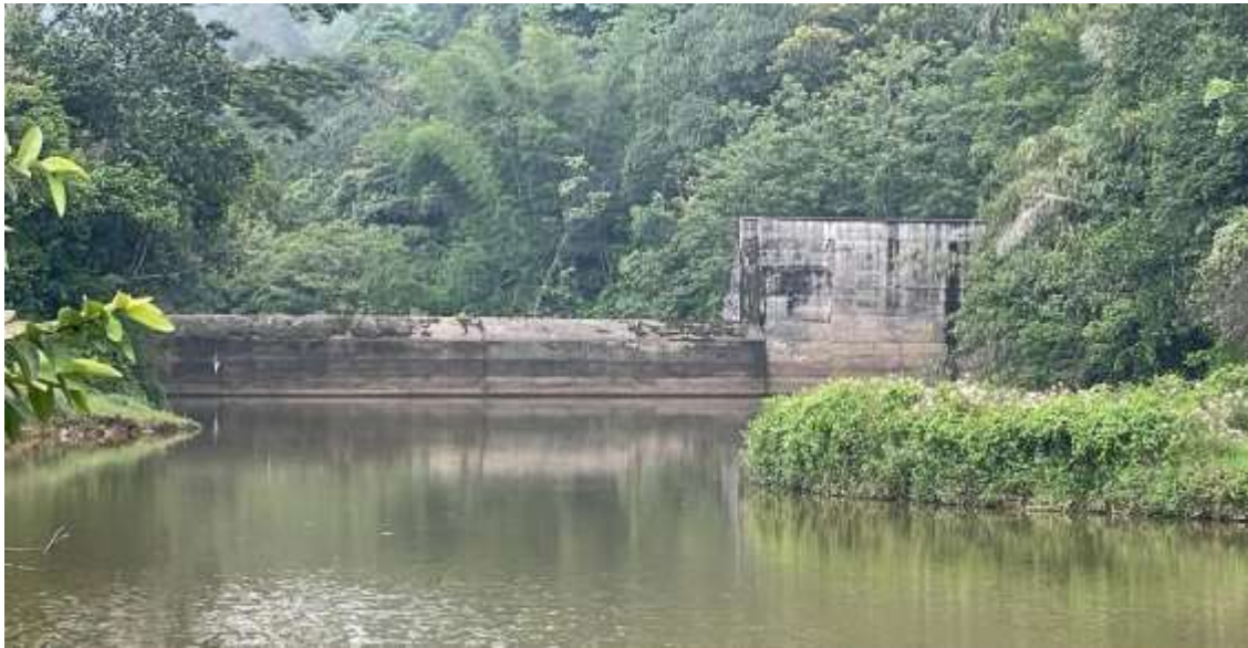
Fig 1.7 Kuttiyar Diversion Weir – Photograph
